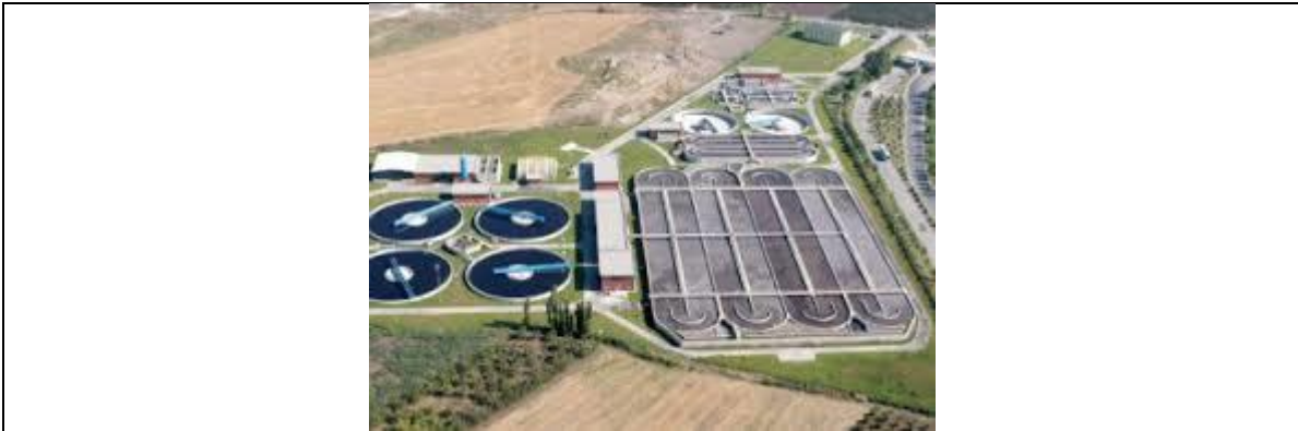
Sewage Disposal (BAİBÜ, Turkey)
