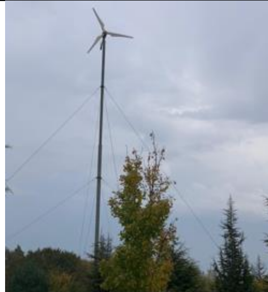
4. Wind Turbine at Gököy Campus (BAİBU, Turkey)
