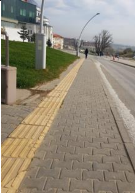
Example of pedestrian path for disabled person at Gol koy Campus (Bolu Abant İzzet Baysal University (BAIBU), Turkey)
