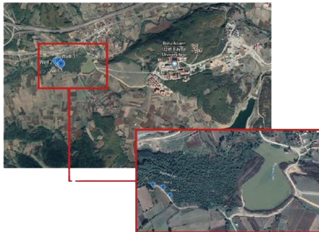
Example of Water Conservation –Wells for Drinking Water Supply at Gököy Campus
