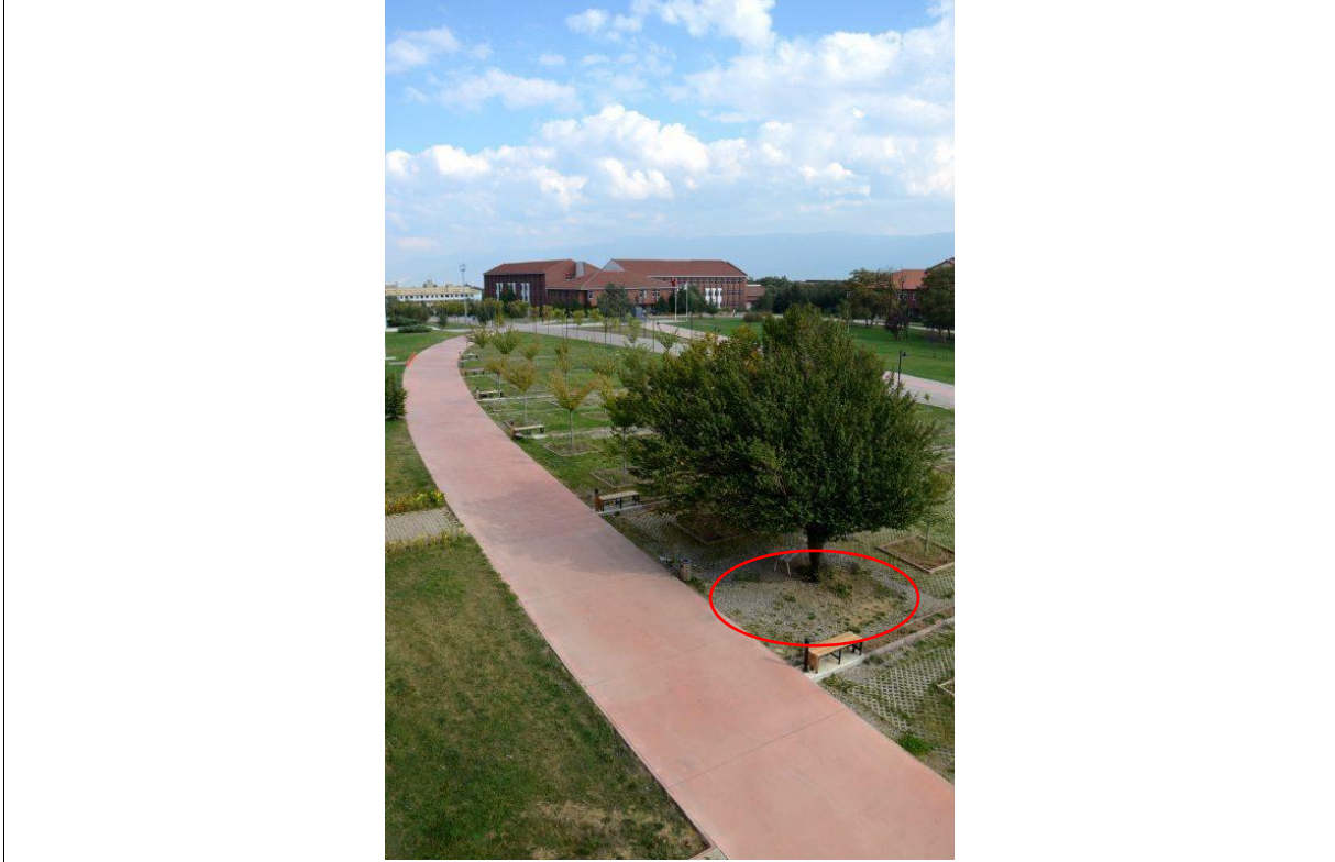
Example of water absorption in Gölköy Campus
