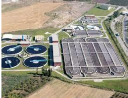
Figure 3.8. Municipal wastewater treatment facility operating in partnership with Bolu Municipality for integrated campus sewage processing.
