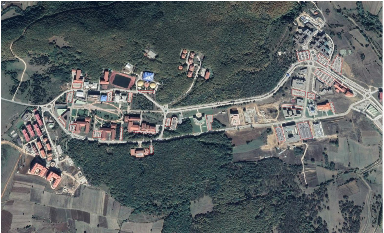
Figure 5.7. Aerial geospatial mapping and infrastructural layout analyzing the distribution of designated parking zones across the Gököy Campus perimeter.
