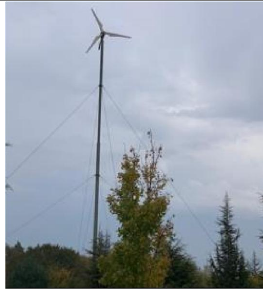
4. Wind Turbine at Gölköy Campus (BAIBU, Türkiye)
