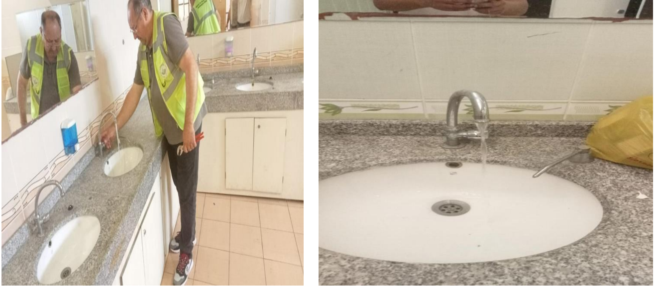
Figure 4.5. Maintenance of water fixtures by technical staff at Gölköy Campus.
