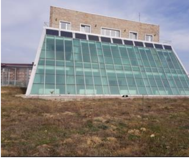
1. Façade Mounted Solar Panels at Gölköy Campus (BAIBU, Türkiye)
